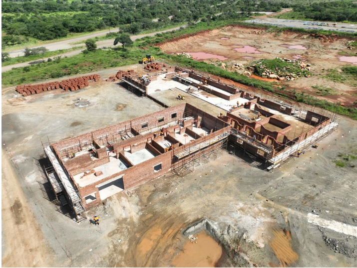
Laboratory Brickwork Construction
