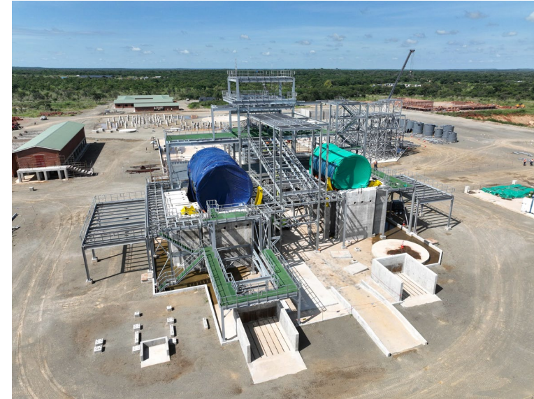
Mill Building Steel Erection
